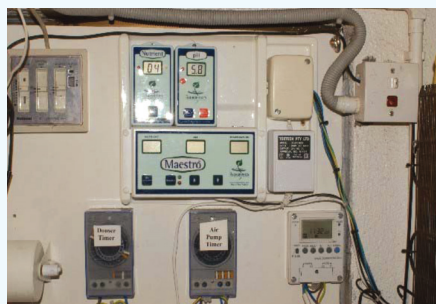
Fig. 2: pH value and nutrient level electronic sensors and regulators
